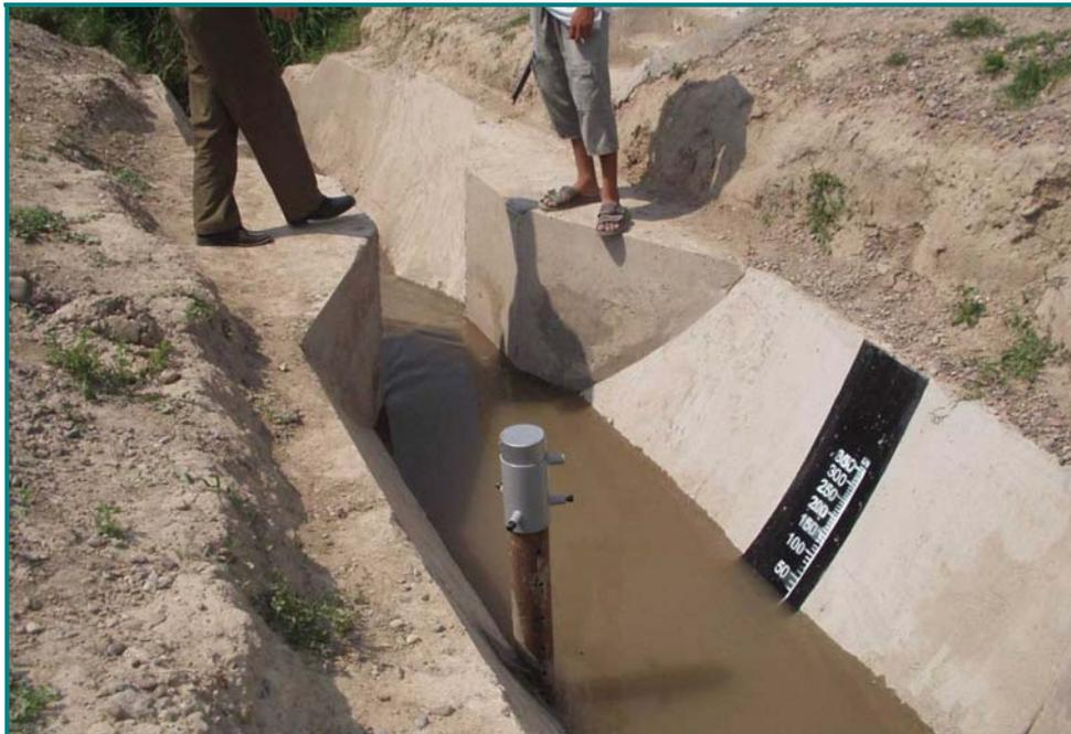
**Picture 4. Sensor on parabolic flume**
